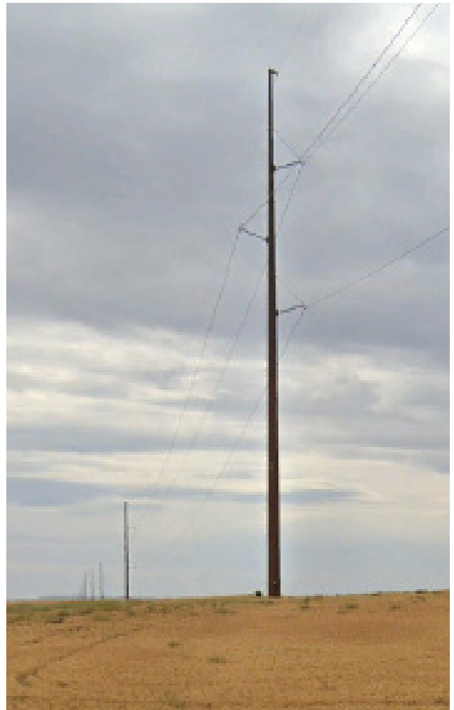
Proposed transmission line structures will look similar to the above photograph.
