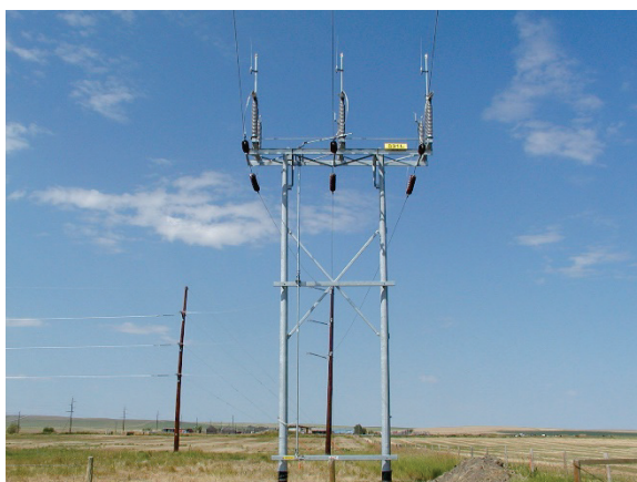
A steel H-frame structure with airbreak similar to those proposed for the project.
