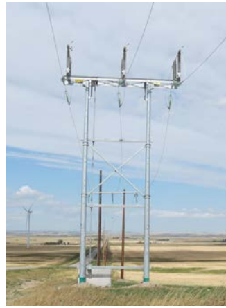
Airbreak steel structure similar to the proposed
