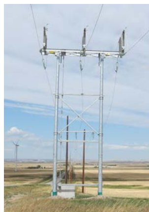
Steel airbreak structure
