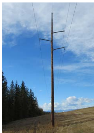
Single pole wood structure
