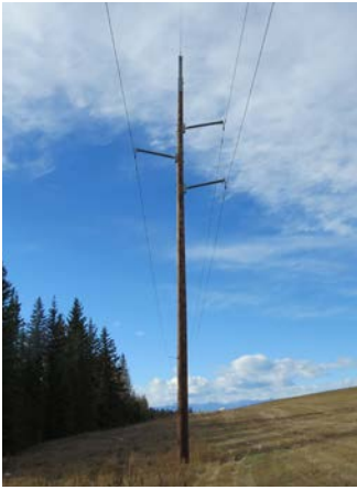
Single pole wood structure similar to the proposed
