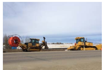
Above: Fibre optic cable being buried. You may see similar construction activities in your area.
