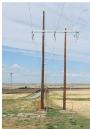
H-frame wood structure
