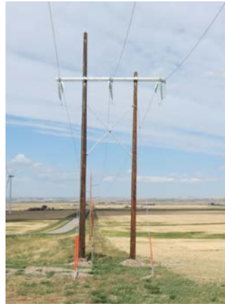
H-frame wood structure similar to the proposed
