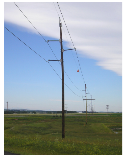
Above: typical three-pole configuration
