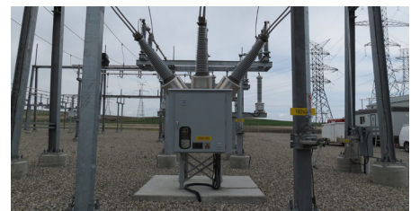
A typical 138 kV circuit breaker
