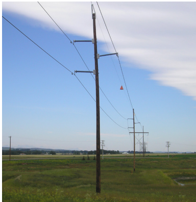
Structures on the new transmission line will look similar to the above
