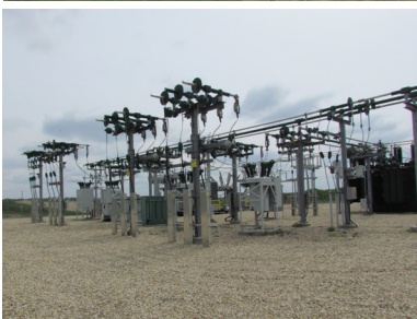
Above: the Provost Substation Middle: the Edgerton Substation Below: the Hayter Substation
