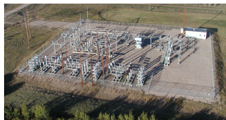
The Killarney Lake Substation
