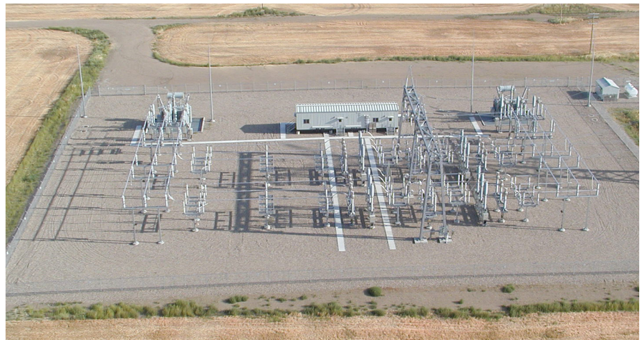
The existing Whitla Substation
