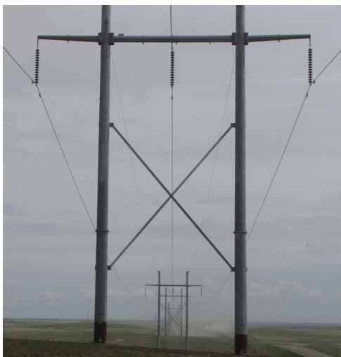
Steel H-frame structure
