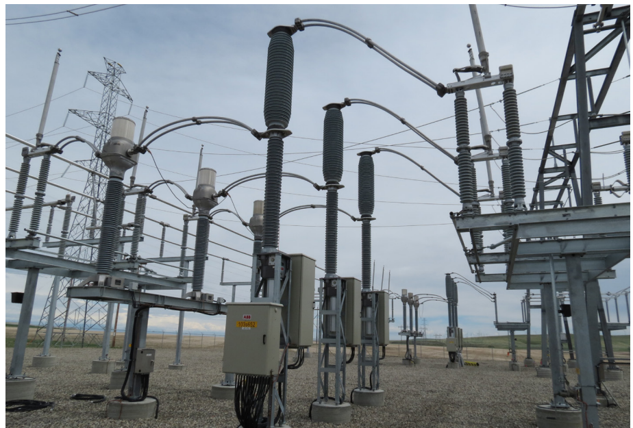
A typical 240 kV circuit breaker
