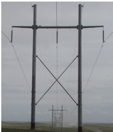
Two-pole H-frame steel structure similar to the proposed
