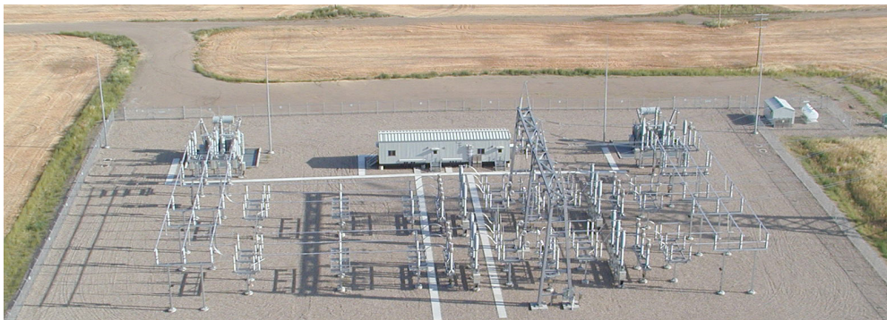
The existing Whitla Substation
