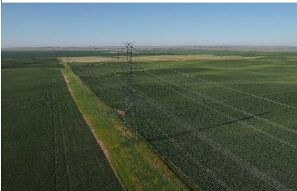
Top: The existing 1005L
