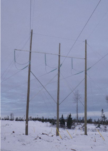
Example H-frame Wood Structure
