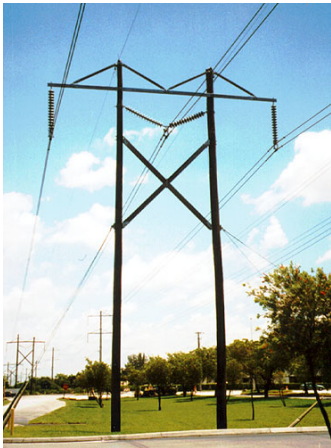
Example H-frame Wood Structure
