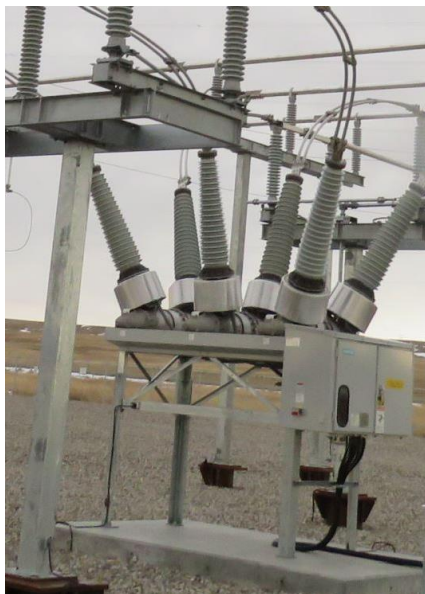
Above: typical 240/138 kV transformer Below: typical 138 kV circuit breaker
