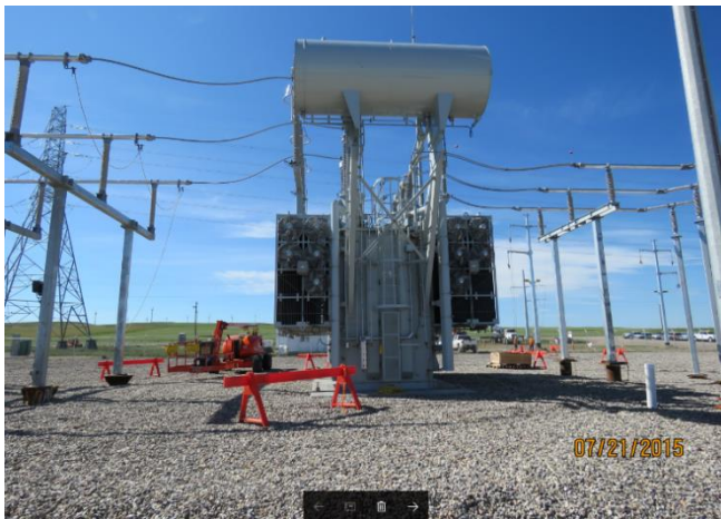
Above: typical 240/138 kV transformer Below: typical 138 kV circuit breaker
