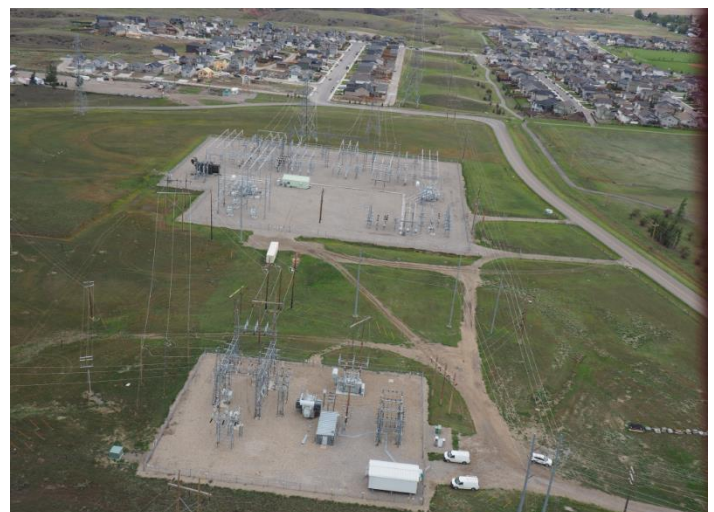
Above: the North Lethbridge Substation
