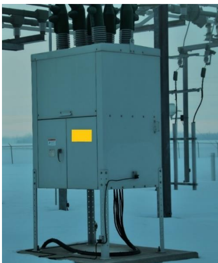
Below: typical 25 kV circuit breaker
