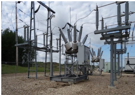
Above: typical 138 kV circuit breaker
