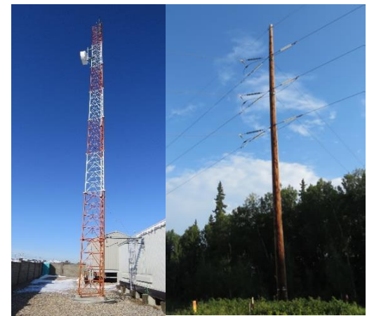
Left: The new telecommunications tower will look similar to the one above
